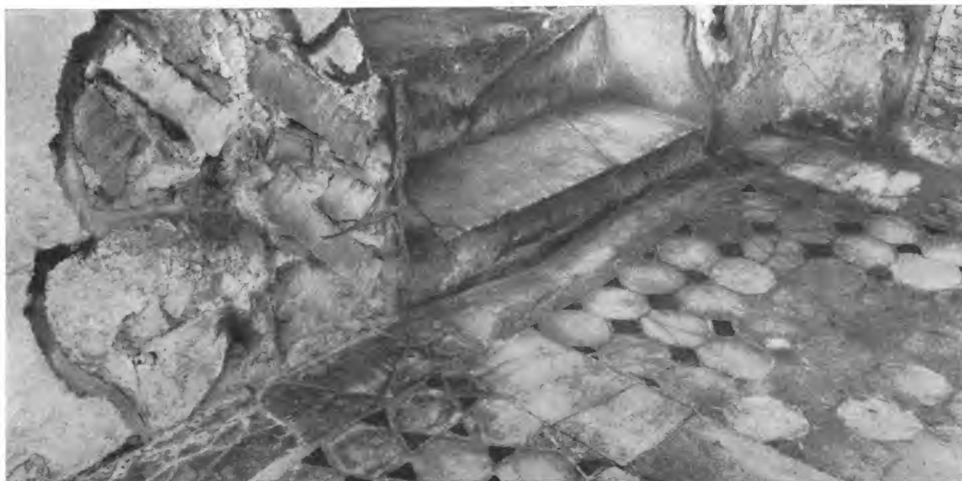
Fig. 202 — S. Maria Antiqua. Opus alexandrinum and opus testaceum at the north-west corner of the tablinum (Photo: Corbett).
